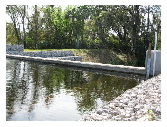
Figure 1-6. Diversion Weir/Overflow Spillway.
