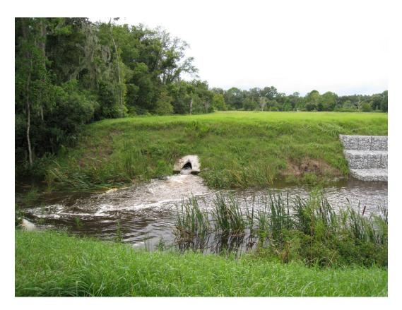
Figure 1-7. Pond Outfall through 24-inch RCP.
