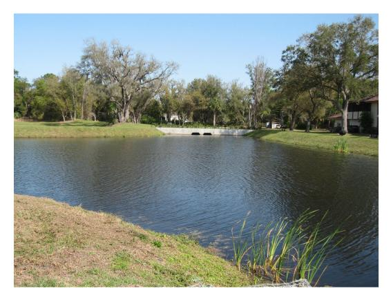
Figure 1-5. Box Culvert Inflows to Treatment Pond.
